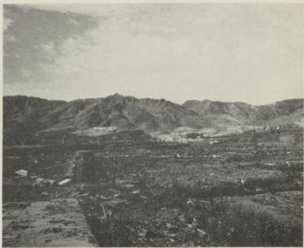
Photo 3. 1500 feet northeast of GZ. Blast and fire damage. Looking southwest.
